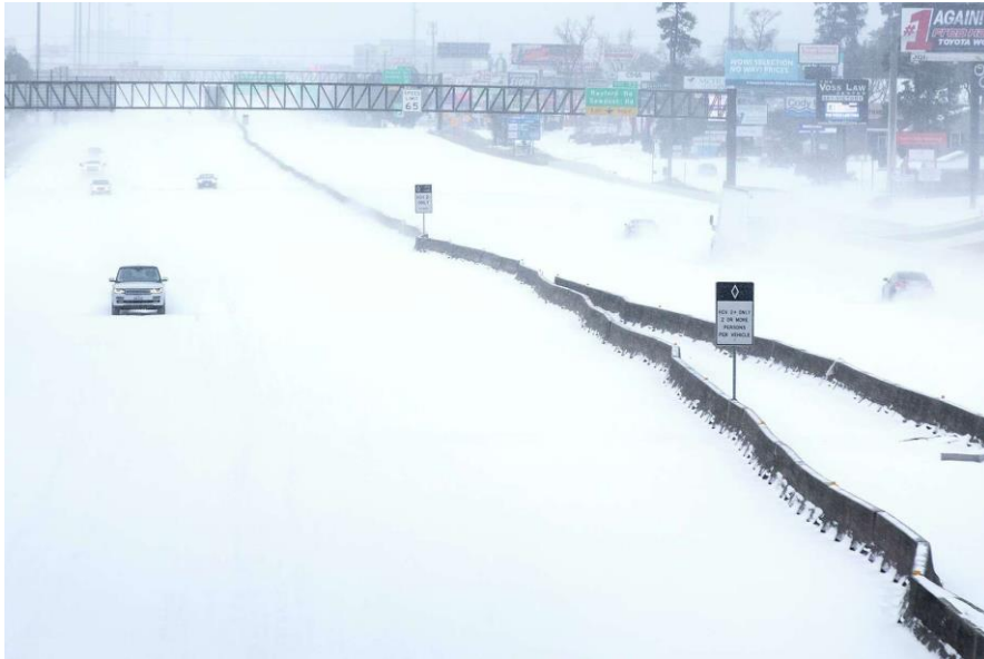
Fig. 9: Texas Deep Freeze of 2021 14 ; Natural disasters affect major highway arteries which if obstructed, prevents people from day-to-day tasks such as grocery store trips, which due to greater distances between destinations, can only comfortably be reached by car
