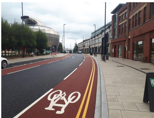
Figure 14: Red-dyed asphalt for bicycle lane (Asphalt Industry Alliance, n.a.)
