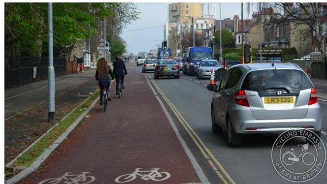
Figure 4: Stepped bicycle path on Hills Road in Cambridge (Cycling Embassy of Great Britain, 2016)
